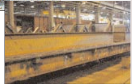
...and retrofitted with a new deck...
